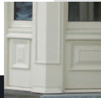
Detail : "Concept III" windows Tilt & Turn Series with decorative rigid aluminum paneling
